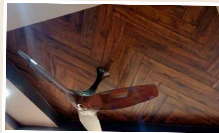
Flooring used in ceiling
