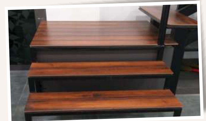
Flooring used in stair case
